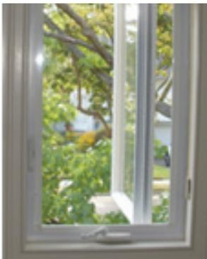
Quality operators allow window to open and close with ease. Fully open casement allows for cleaning from inside.
