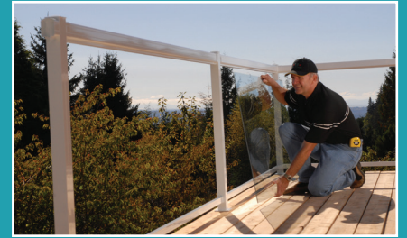
STEP 3: Install Tempered Glass
