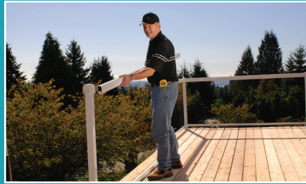
STEP 2: Install Top & Bottom Rails
